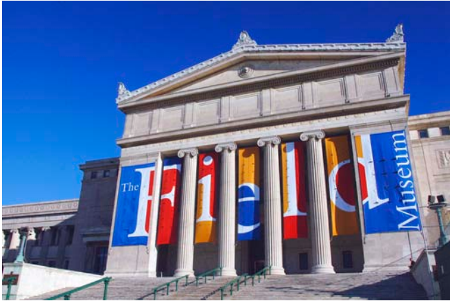
Photo Credit: ©City of Chicago
